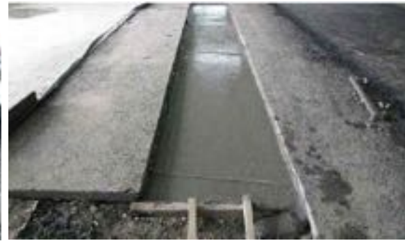
(b) 1 st Concrete layer
