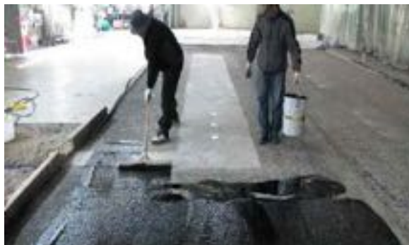
(e) Tack coat
