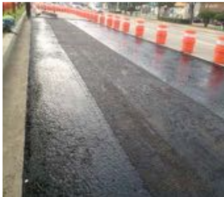
(f) Tack coat and surface layer application
