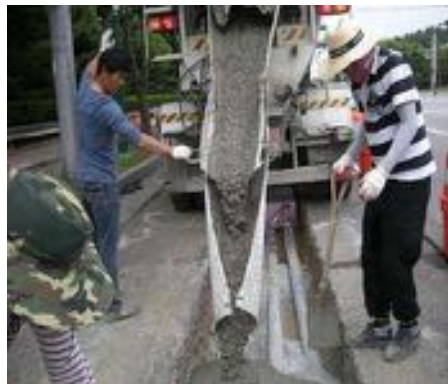
(e) Concrete fill around system
