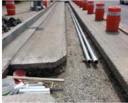
(a) Trench excavation and placement of pipes
