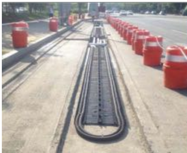
(a) In-situ construction
