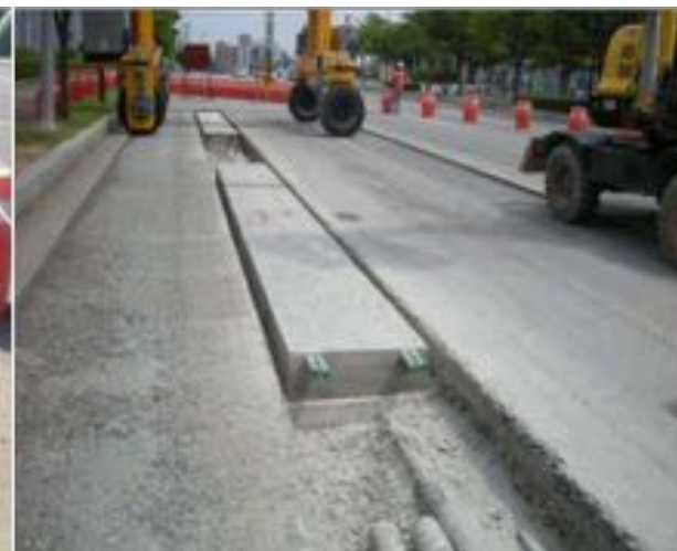
(b) Prefabricated system
