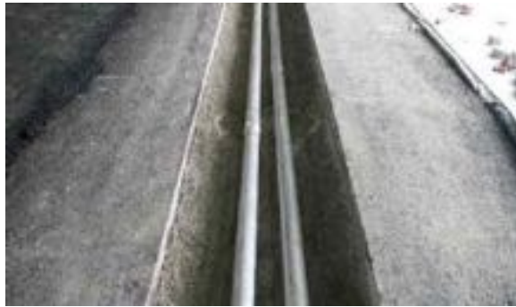
(a) Trench excavation and placement of pipes
