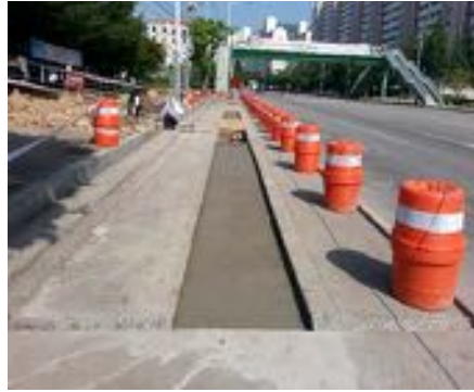
(b) 1 st Concrete layer
