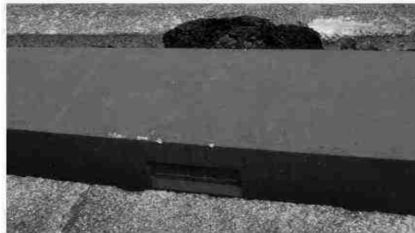
Pre-casting concrete type of power line module
